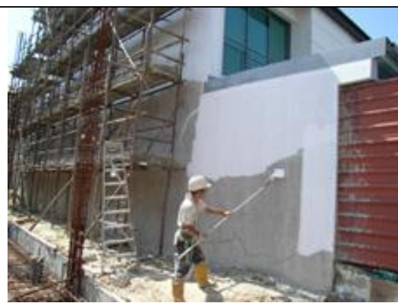
QUICSEAL 103 ECO for external wall waterproofing
