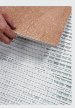
Restoring tiles with an overlay solution is a cost-effective and straightforward way to give a new look to walls and floors in a shorter time. ARDEX products can facilitate the rapid repair of damage to loosened tiles or the replacement of existing ones without the expense of a new installation.
