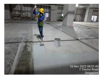
Application of ARDEX BRP 35 EP an epoxy bonding bridge
