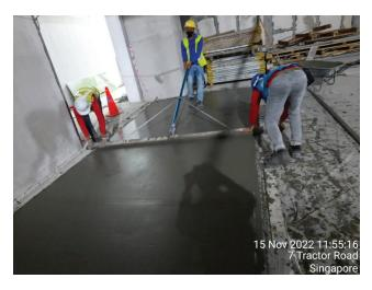
Final levelling to Floor finish level
