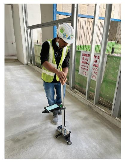
Checking of floor level and flatness to ASTM115E using dip stick
