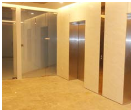
QUICSEAL 602+604 High Flexibility Tile Adhesive (EN Classification: C2TES1) – used to install all the marble and granites in internal and external areas, including large-sized one metre by one metre marble at lift lobbies.
