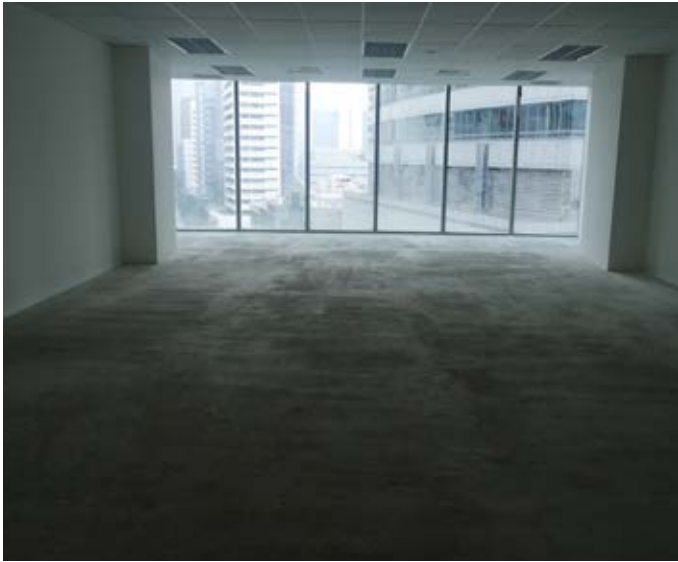
QUICSEAL 534HD High Strength Levelling Screed – used to level the concrete surface for thickness ranging from 10mm to 60mm.
