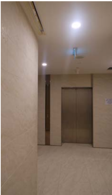
QUICSEAL 601 High Strength Tile Adhesive (EN Classification: C2TE) – used to install homogenous tiles at lift lobbies and common toilets.
