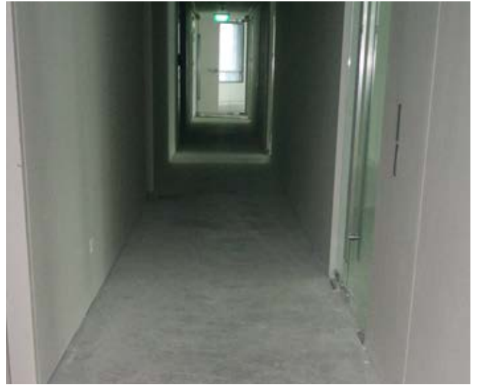
QUICSEAL 531 Semi-Flowable Levelling Screed – used to level the concrete surface for thickness ranging from 3mm to 6mm.
