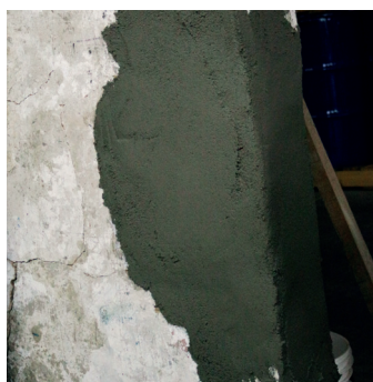
8 Smoothen the repaired area to achieve the desired finish
