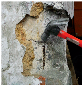
2 Hack out weak or carbonated concrete until sound concrete is detected
