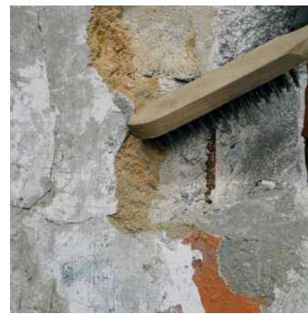
3 Use a wire brush to remove rust from the reinforcement
