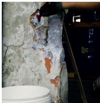
5 Use a brush to prime the substrate with QUICSEAL 607 Easi-Bond SBR latex admixture
