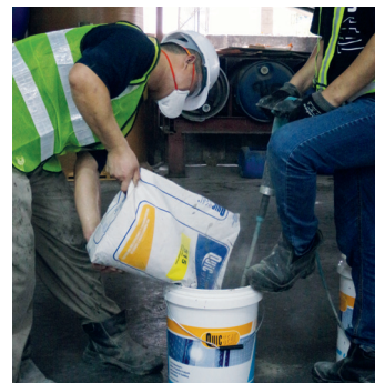
6 Mix QUICSEAL 515 repair mortar with water until a homogenous paste is obtained
