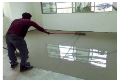
QUICSEAL 571 spread evenly using a spiked roller.
