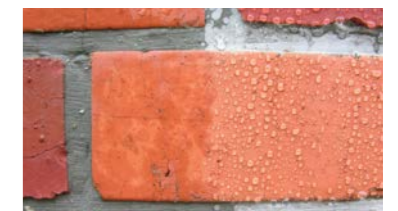
QUICSEAL 110 impregnator used to treat brickwork finishes.
