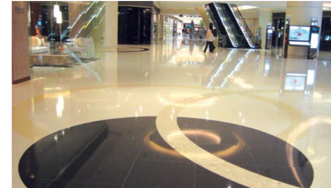
QUICSEAL 615 and 532 fast set adhesive and screed used for upgrading works.
