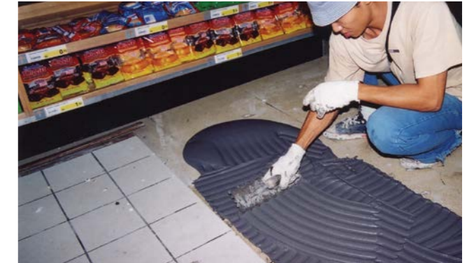
QUICSEAL 685 fast set adhesive used for quick tile installation.
