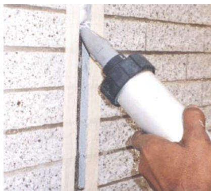
QUICSEAL 210 Modified Silicone sealant used for movement joints on natural stone facades (non-staining).
