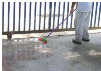
QUICSEAL 538 liquid floor hardener for old concrete surface.
