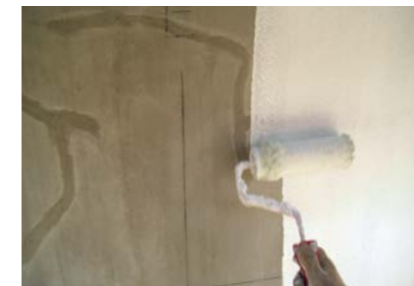
External Wall Seepage Repair System QUICSEAL 304 epoxy putty. QUICSEAL 103M acrylic waterproofing coating.
