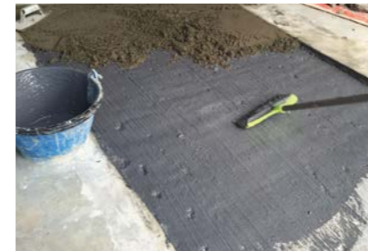
QUICSEAL 534HD (heavy duty) levelling screed up to 60mm with QUICSEAL 607 latex as slurry bond coat.
