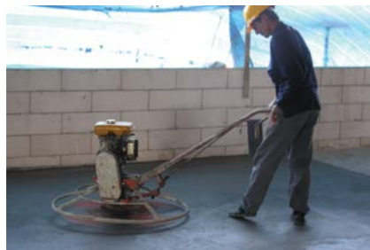
QUICSEAL 535 monolithic floor hardener for new concrete flooring.
