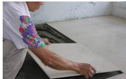
QUICSEAL 601 single component polymer modified adhesive used for large porcelain tile installation.
