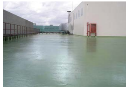
QUICSEAL 161 PU system used for waterproofing M&E roofs.
