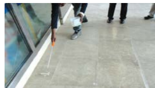
Treatment of tiles using QUICSEAL 651 Q-Cleaner.
