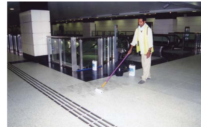
QUICSEAL 630 / QUICSEAL 632 oil and water repellent impregnator protects granite and marble finishes against staining.
