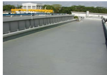
QUICSEAL 161 UV resistant PU waterproofing system for RC flat roofs.
