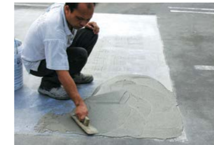
Carpark & Repair System QUICSEAL 113 primer / QUICSEAL 607 bonding agent. QUICSEAL 531 for carpark patch repair and resurfacing.
