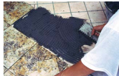
QUICSEAL 604/602 used for tile-on-tile installation.
