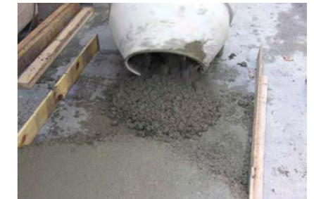
QUICSEAL 532HD (heavy duty) fast set screed top up for carpark and heavy trafficking areas.
