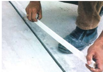
QUICSEAL 401 crack inducer and movement joint former.
