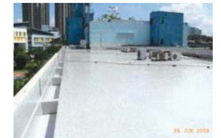
RC Roof Seepage Repair System QUICSEAL 304 epoxy putty. QUICSEAL 161 waterproofing membrane.
