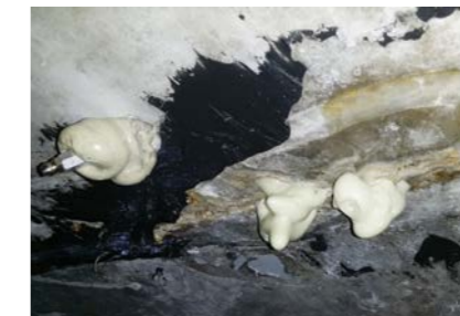
QUICSEAL 172 PU injection resin to stop water ingress.
