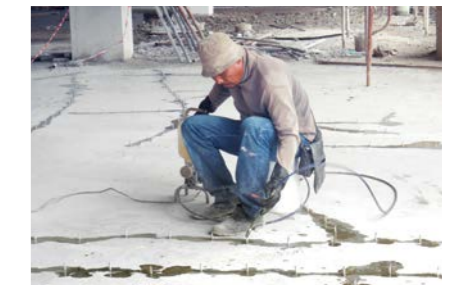
QUICSEAL 302LV for structural crack repair under damp condition.
