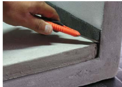
QUICSEAL 406 joint filler used for perimeter joints.
