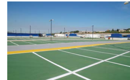
QUICSEAL 161 & 372 polyurethane system for exposed carpark decks.
