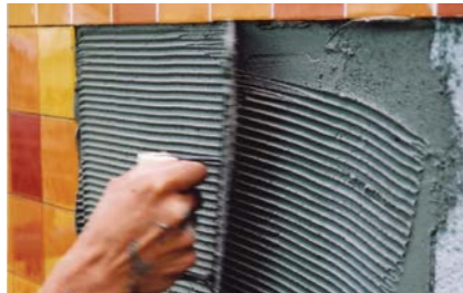
QUICSEAL 600 cement based adhesive for ceramic tile installation.
