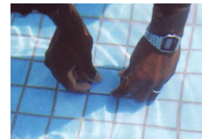
QUICSEAL 301 for underwater tiles bonding repairs.
