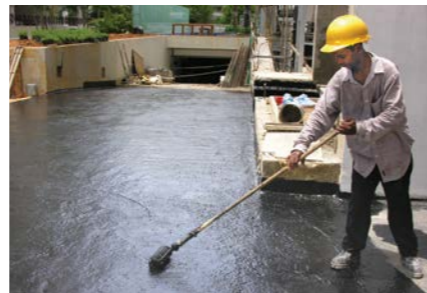
QUICSEAL 102 : Single Component, ready-to-use, liquid applied waterproof membrane.
