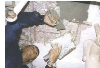
Spalling Concrete Repair System QUICSEAL 504 rust protector. QUICSEAL 607 bonding agent. QUICSEAL 514 repair mortar.
