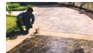
QUICSEAL 107HD sealer used or sealing slate tiles.
