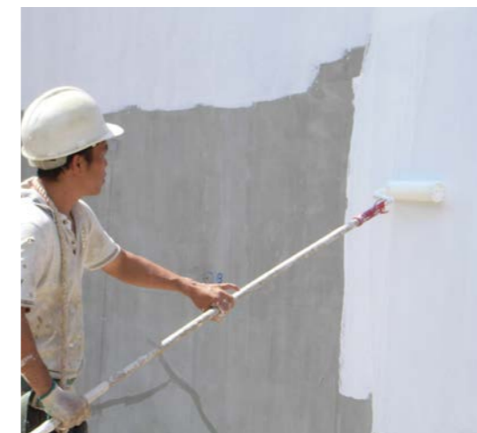
QUICSEAL 103 / QUICSEAL 103 ECO single component, liquid applied, water-based acrylic waterproofing membrane for waterproofing treatment & seepage repairs to external wall.
