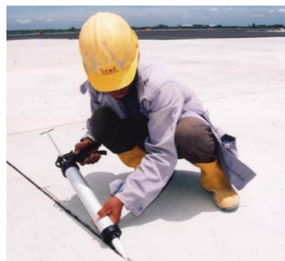
QUICSEAL 208 polysulphide sealant for rigid pavements / QUICSEAL 200 jet fuel resistant, polyurethane sealant for runways.
